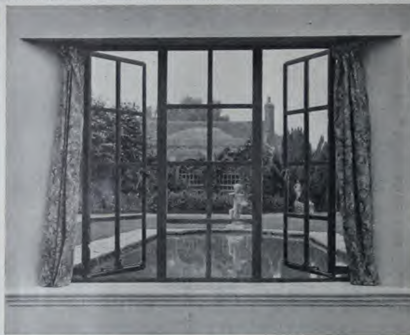
INTERIOR VIEW OF V.8. WINDOW SHEWING HOPE'S SPECIAL CLEANING HINGES
